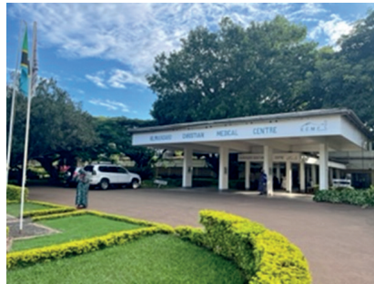
KCMC main entrance.
